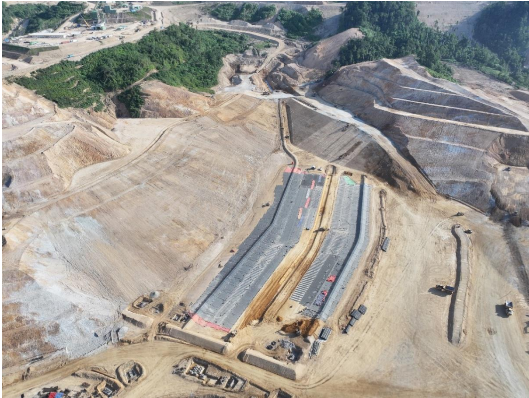
Figure 2: Heap Leach Pad Cell #1, Bay 1 and Bay 2
