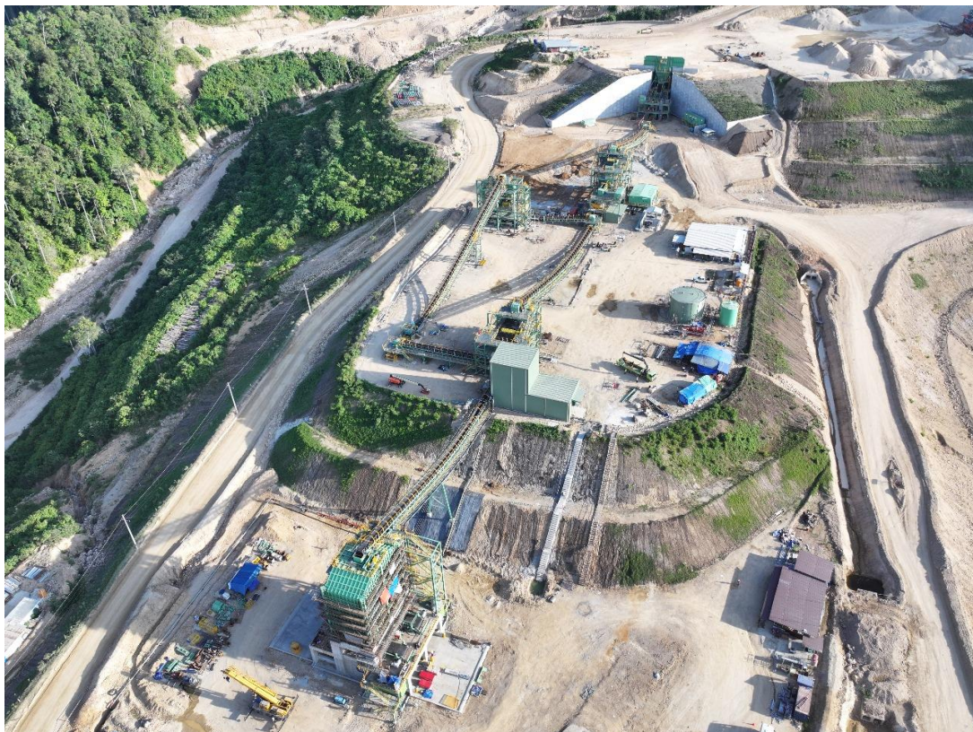
Figure 3: Ore processing plant construction
